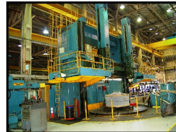
Morando VBM Rebuild & Retrofit
